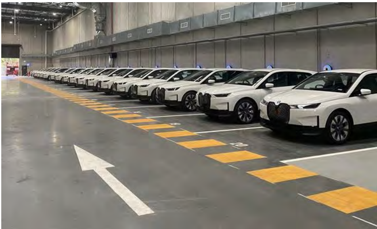
COMCAR's electric vehicle fleet and charging facility located in Melbourne.
