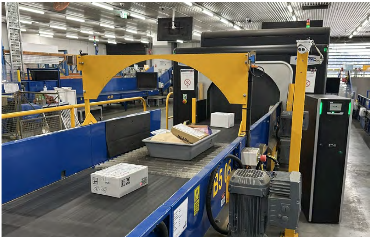
International Mail Inspection at the Australia Post Melbourne Gateway Facility.
